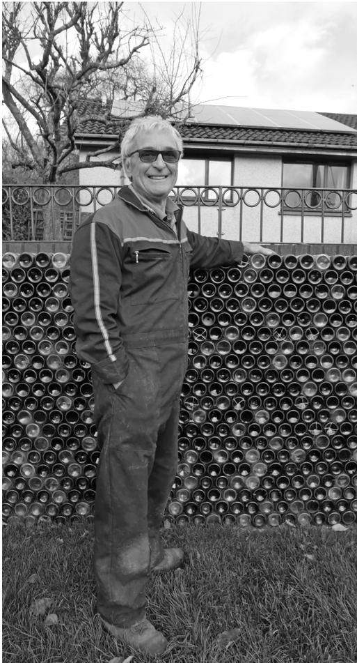
A plan was hatched. It would be a retaining wall 1.4metres high (1.9 to the pillars) and 7.9 long and strong enough to hold back many tons of earth. Footings were dug, concrete poured and blocks were laid flat to form the main body of wall. A hidden buttress midway and behind gives additional support. None of this is seen.
